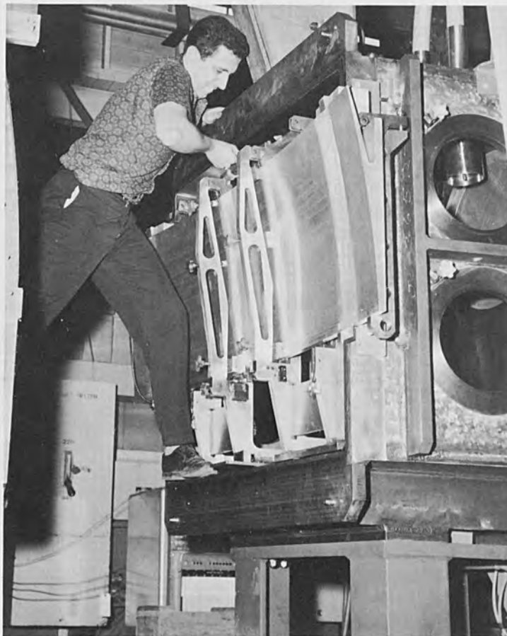
Fig. 17. Y-ring electron-beam welder. Chamber shown open with curved Y-ring section being set in place for welding.
