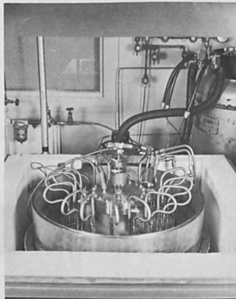
Figure 3. E/B Furnace in Bakeout Oven
