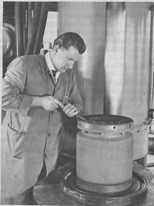
Figure 4. Cleaning of Crucible.
