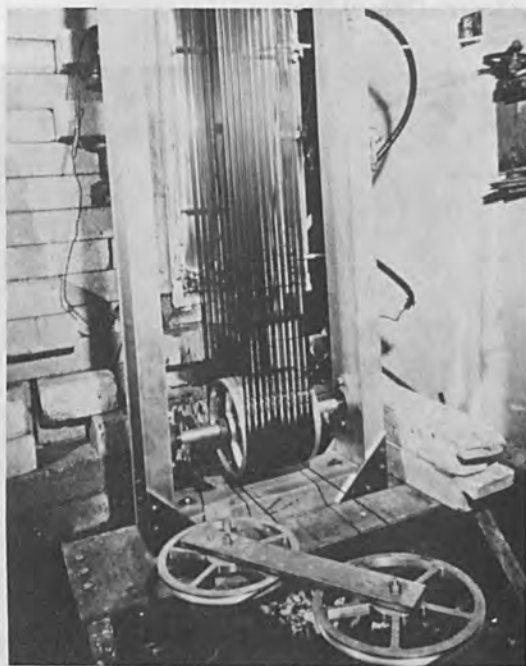
Figure 2. Dynamitron Facility for Irradiation of Plastic Tubing (Radiation Dynamics, Inc.).
