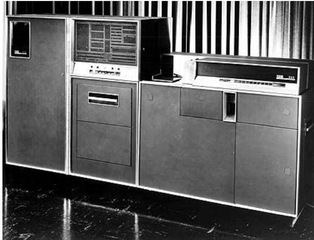
Figure. 1 The IBM 608 computer, first introduced in 1955, was hot technology at the first Beams meeting. It was the first commercial computer to be completely transistorized (no vacuum tubes!!). It contained a whopping 3000 tiny germanium transistors, each about the size of a paper clip and individually soldered. It could perform more than 4000 additions per second! The machine could store up to 40 nine-digit numbers and programs containing up to 80 steps! Data input from punch cards could be processed at a blazing speed of 155 cards/minute! Retail price in 1957 was a very affordable $83,210. ( http://www-03.ibm.com/ibm/history )
